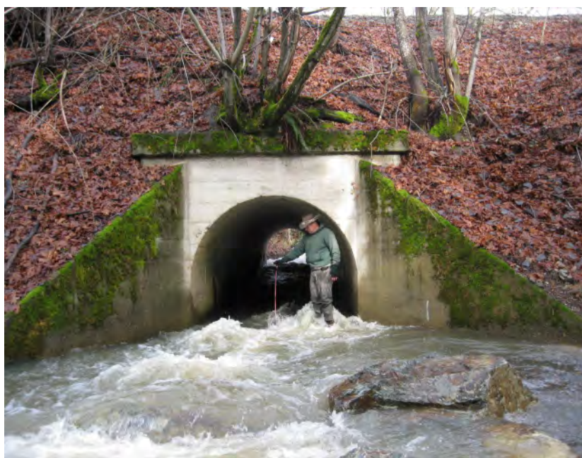
Figure A-I: 3. Railroad culvert on Jones Creek after passage project.
